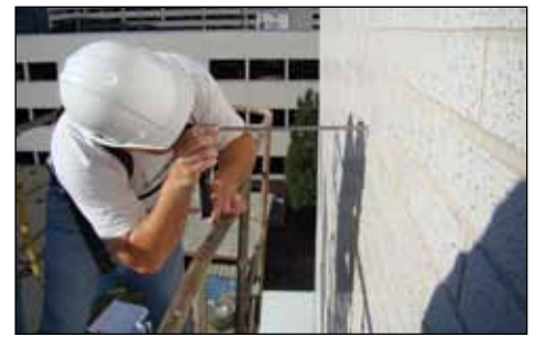
Detailed façade inspection utilizing borescope examination of veneer supports.
