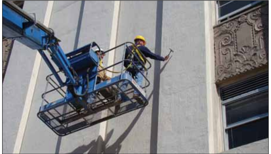
Detailed Façade inspection including sounding for delamination being conducted from a telescoping boom lift.
