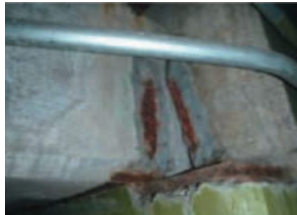
Figure 5 Rebar corrosion and failed repair
