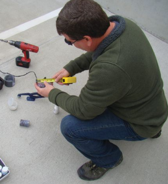
Chloride ion and carbonation testing
