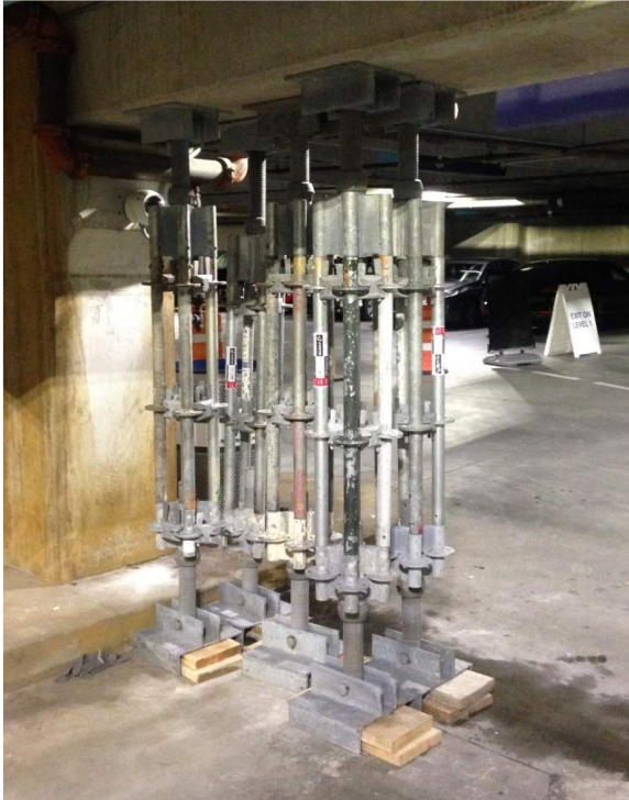
Shoring to Remove Load
