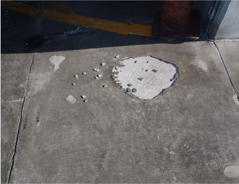
Delaminating Topping
