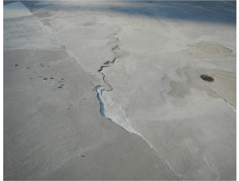
Delaminating Topping
