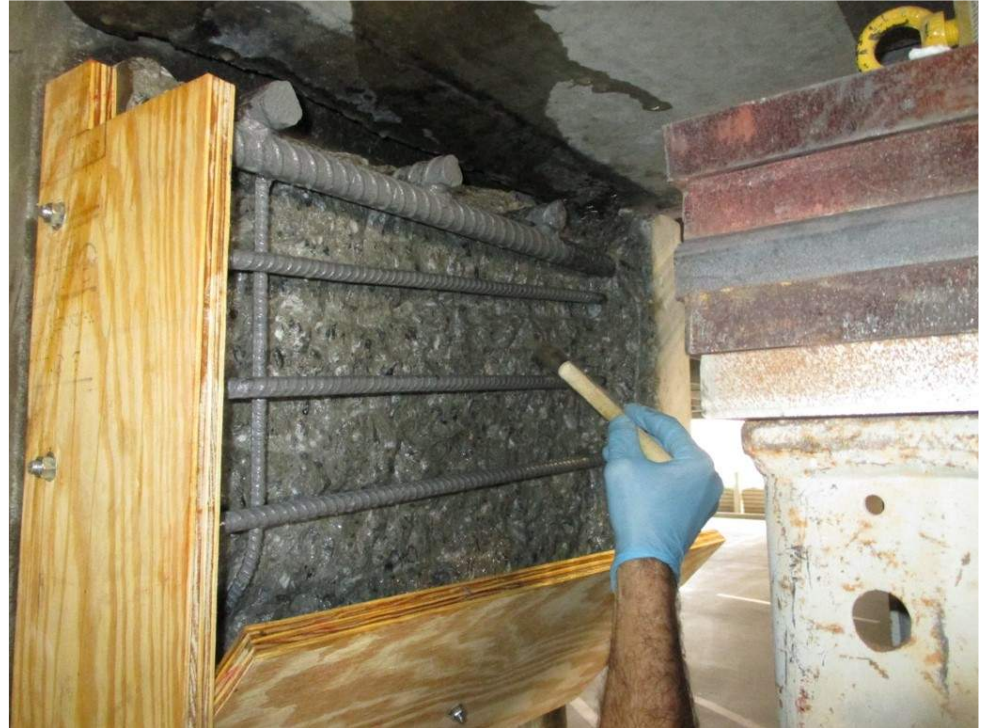
Applying Epoxy Bonding Agent
