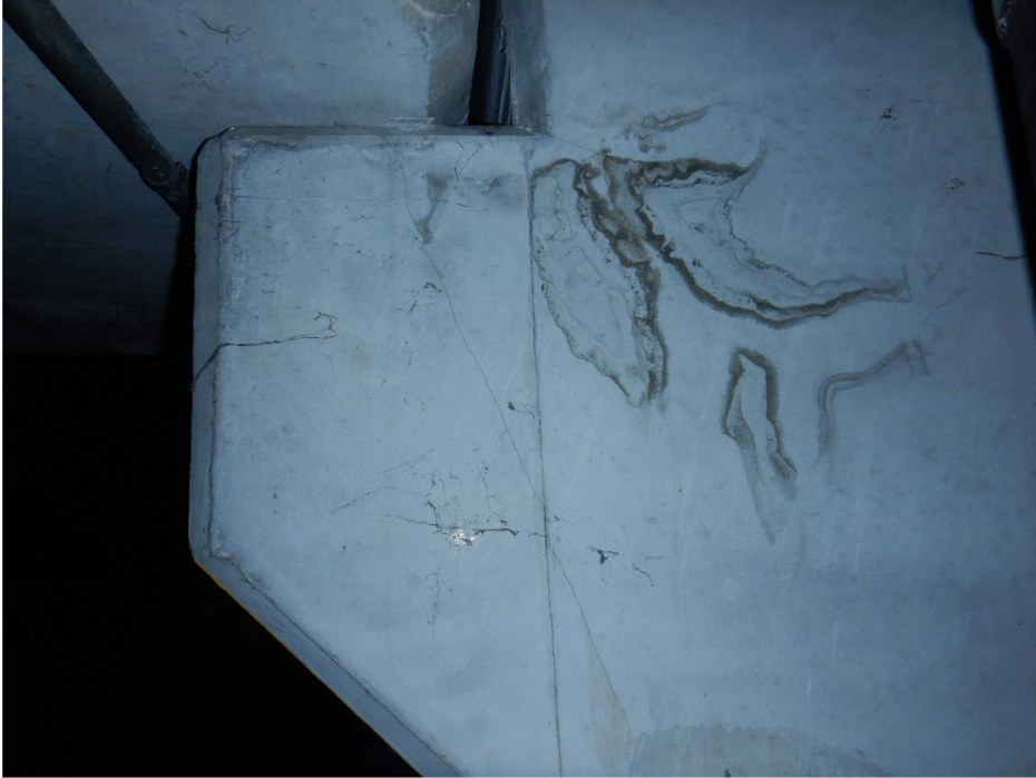
Concrete to Concrete Contact
