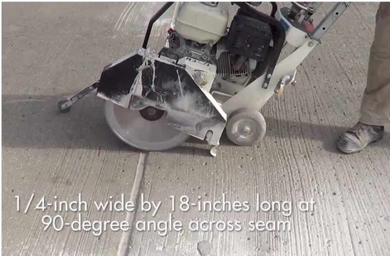
Saw Cut Slab
