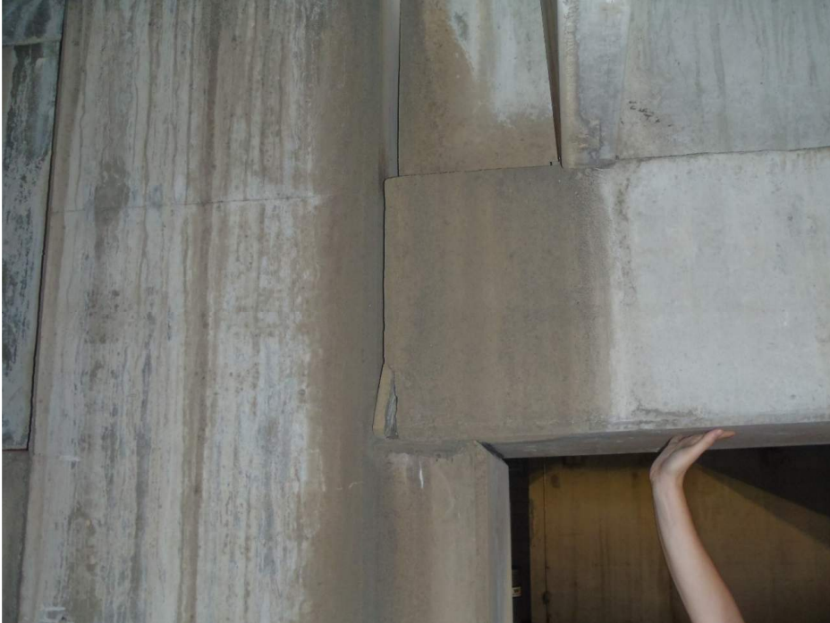
Precast Beam Corbel
