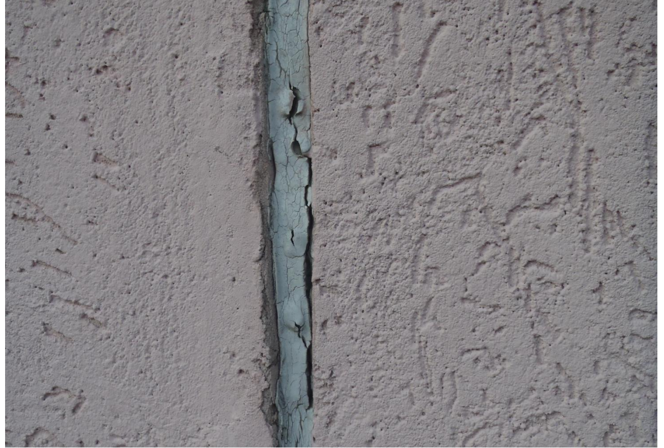
Level B: Failed Sealant
