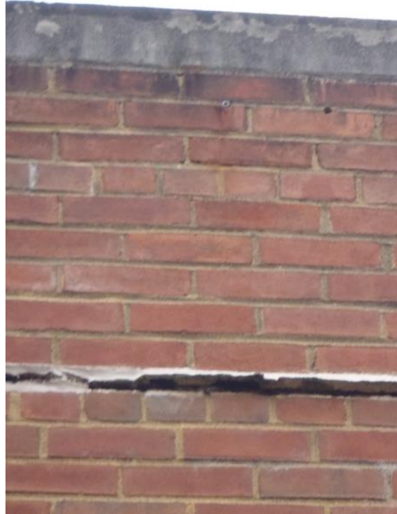
Bond Break at Roof Line
