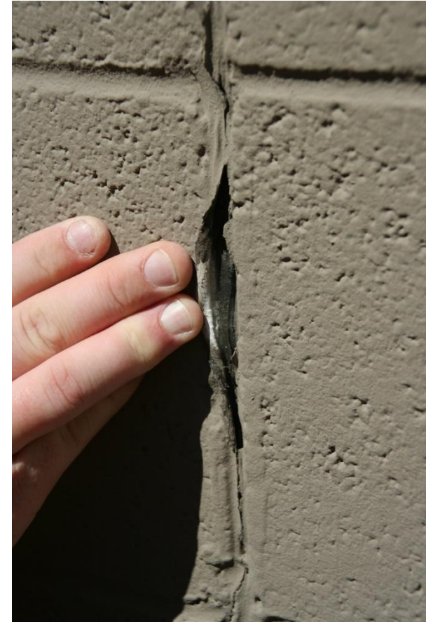
Failed Sealant
