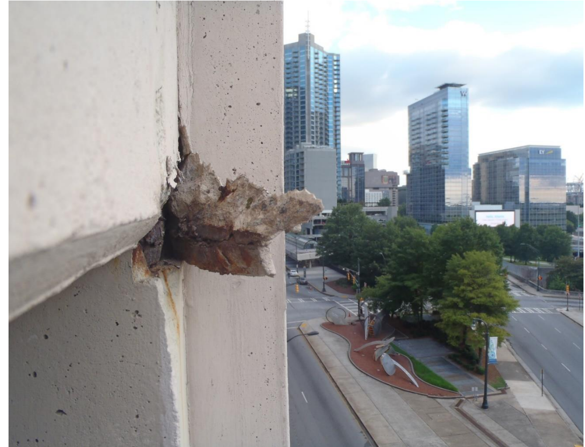
Concrete Spalls
