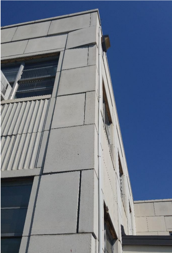
Level D: Loose Stone Panels
